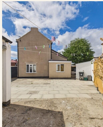
REAR UTILITY AREA
