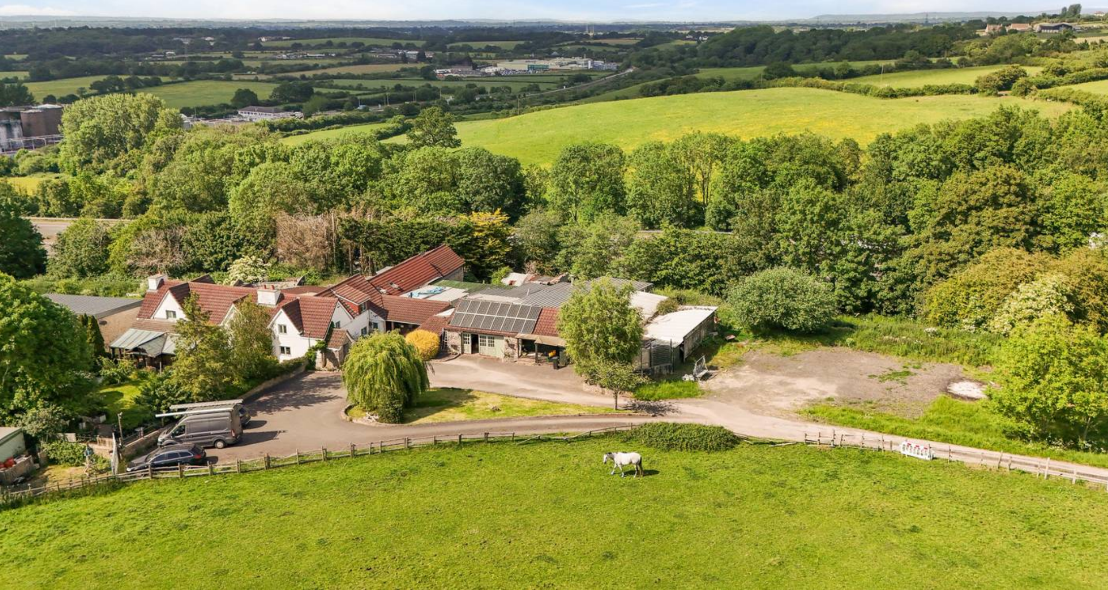
Park Farm House Pucklechurch
