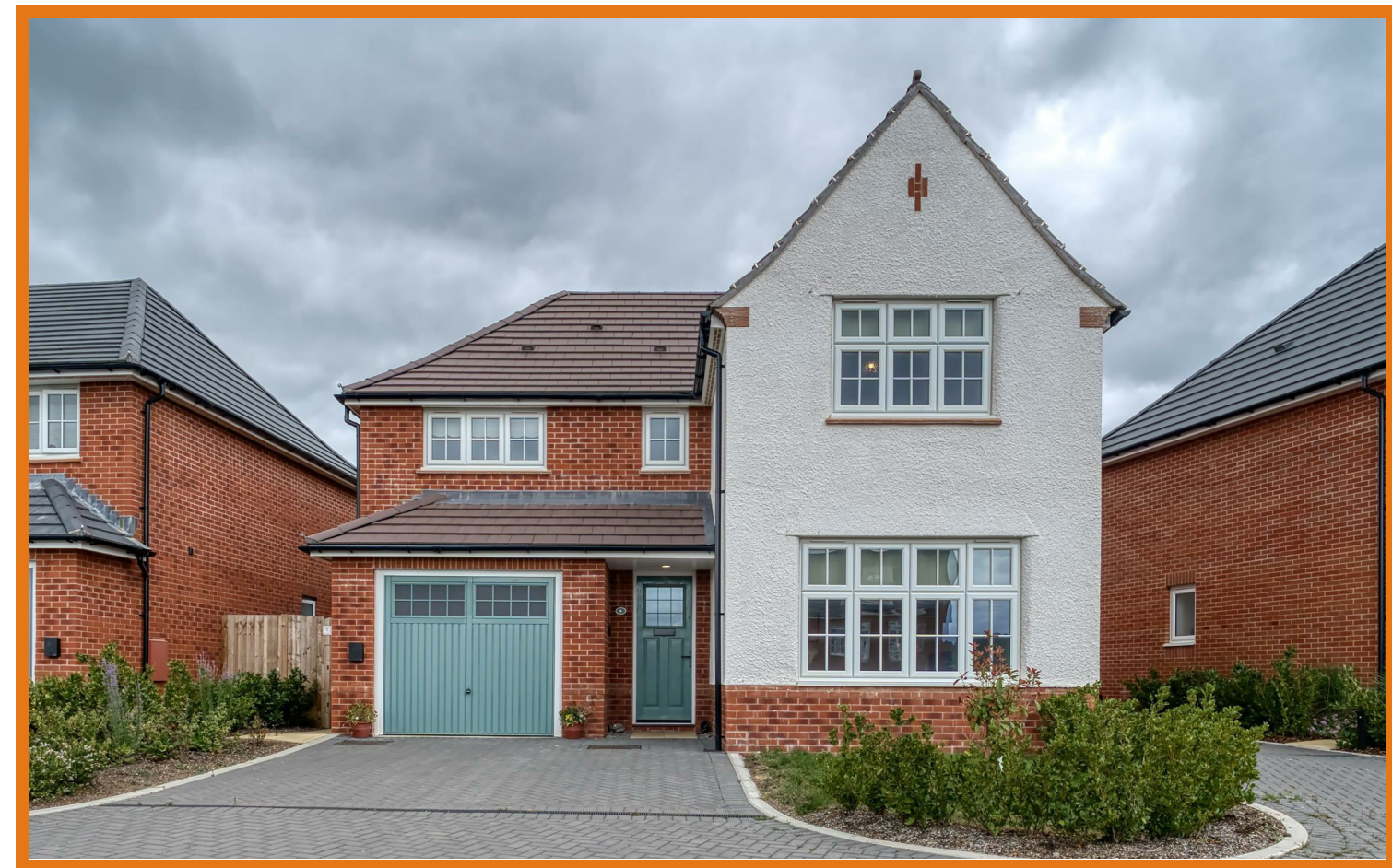
Tile Terrace Gillingham
