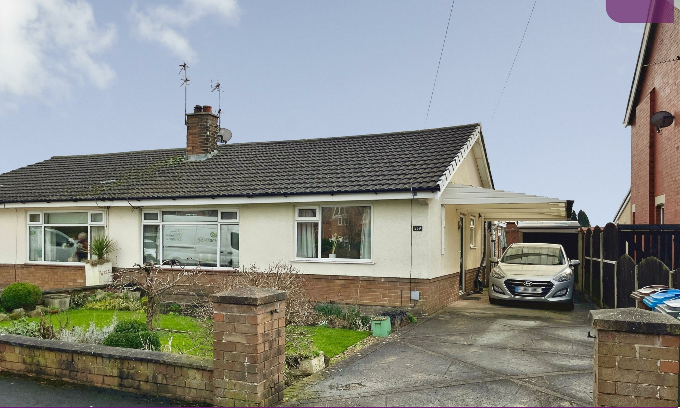
239 Lytham Road, Warton, Preston, PR4 1AE £199,995
