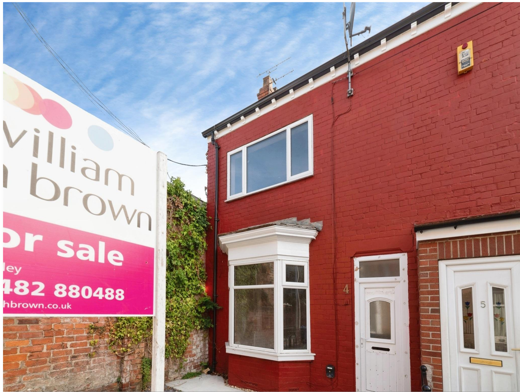
Pretoria Villas, Hull, HU5 2RT
