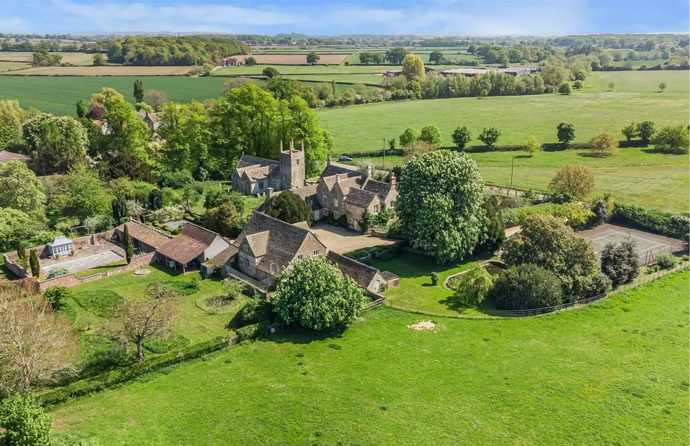
Foxley House - Aerial view looking on to the neighbouring parish church and surrounding countryside
