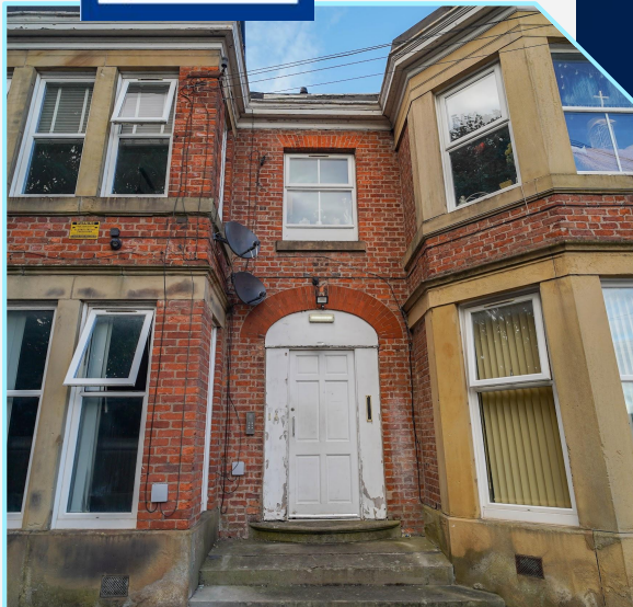
Beechfield House Fourth Avenue M27 5RB
