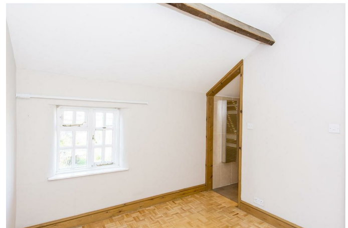
Timber framed double-glazed window to rear. Radiator. Opening through to en-suite shower room.
