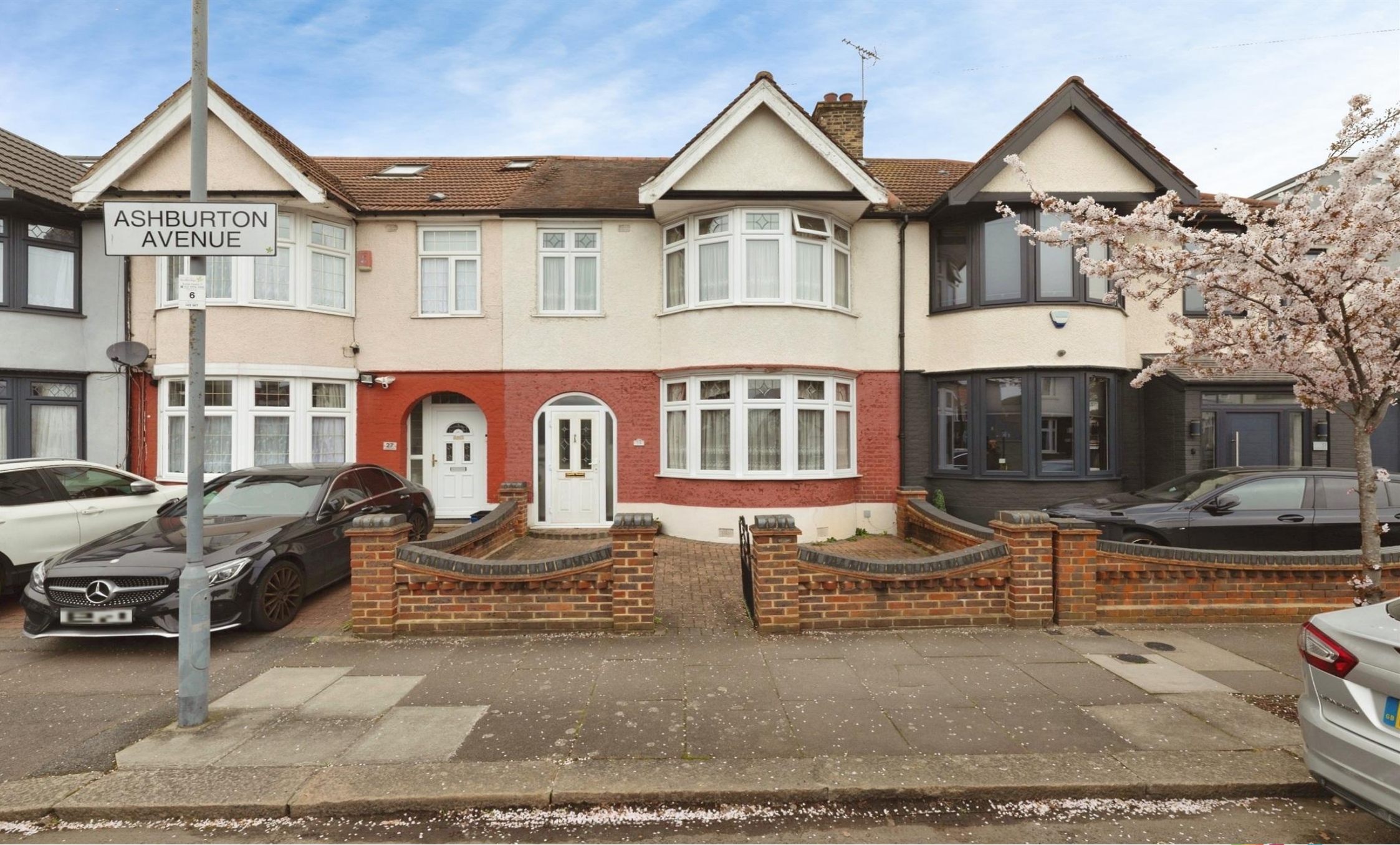
Ashburton Avenue, Ilford, IG3 9ET
