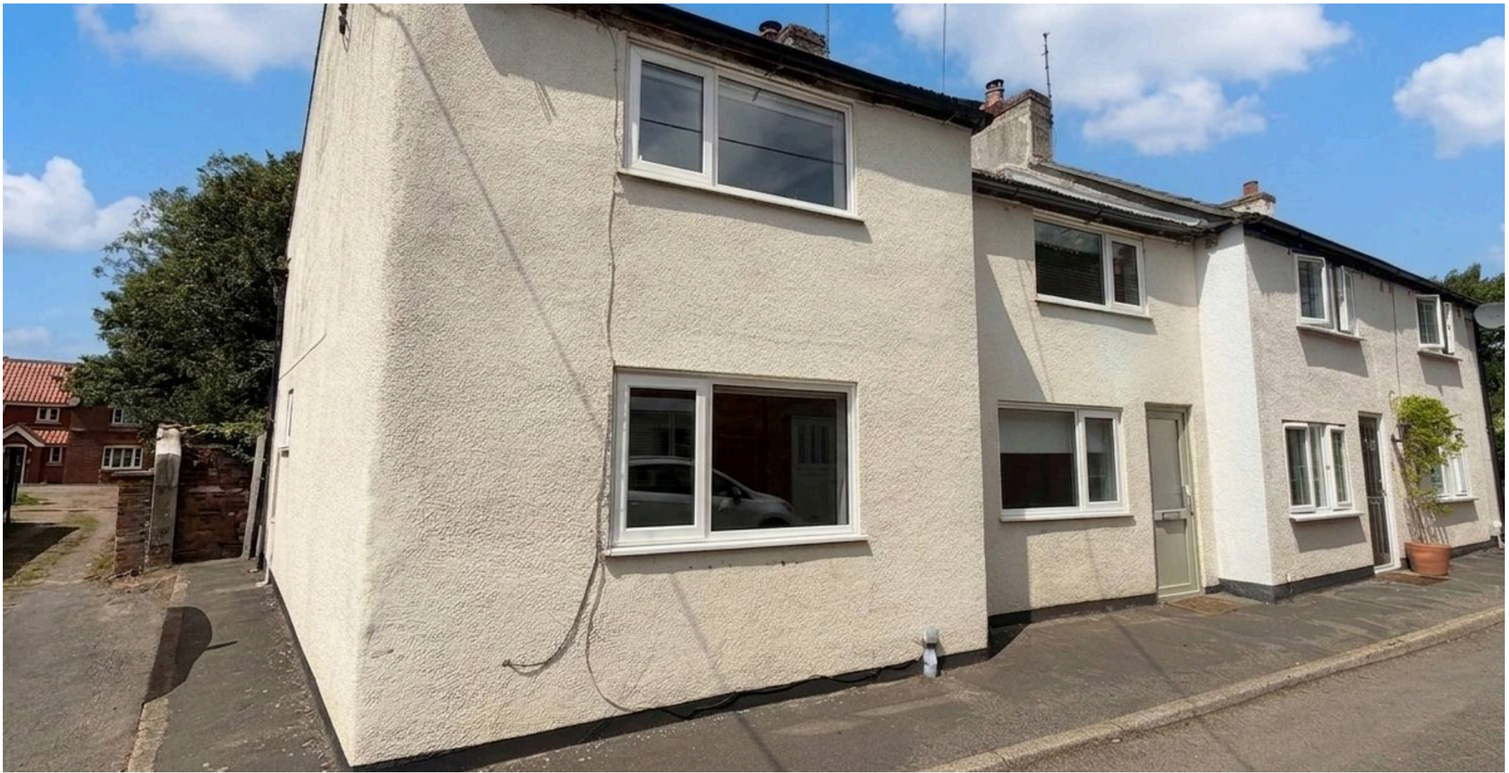
2 Post House Church Street, Barrowby Grantham
