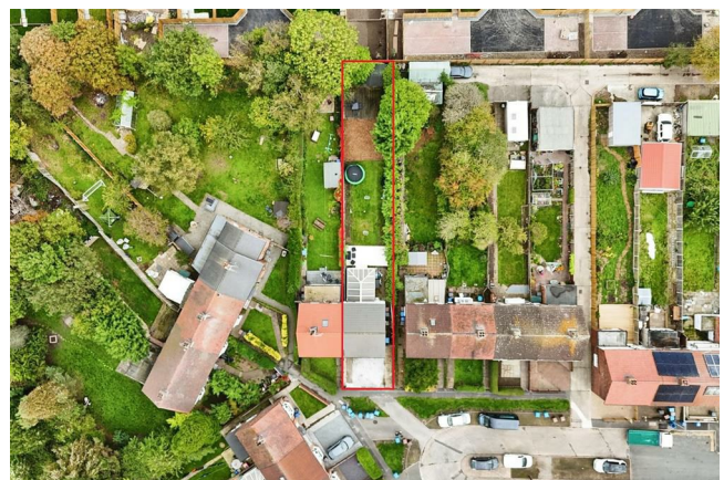
Aerial view of the property
