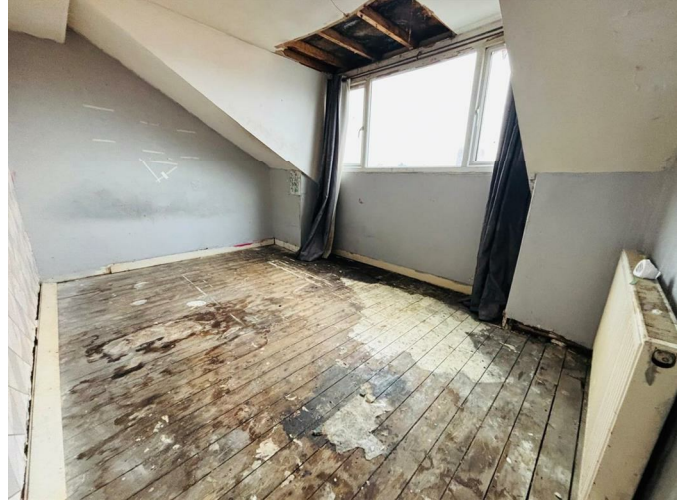
Double glazed window, central heating radiator
