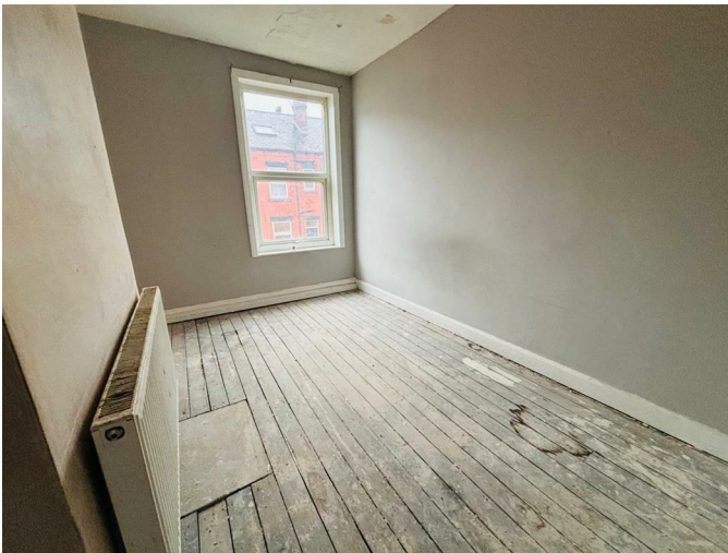
Double glazed window, central heating radiator
