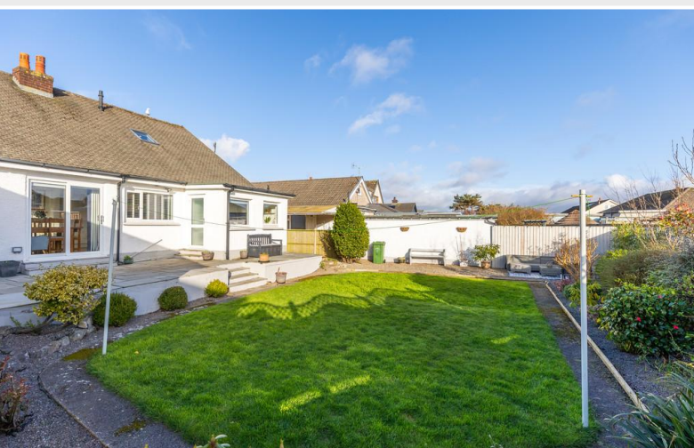
External rear view
