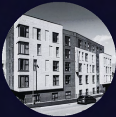
New Bedford House
