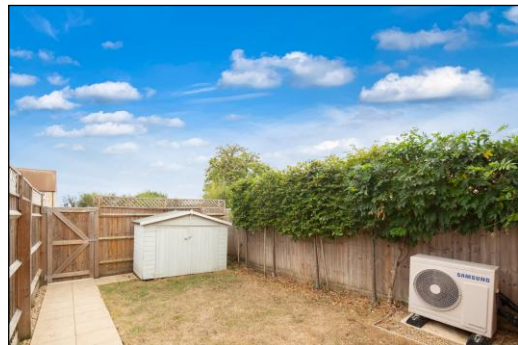
Rear Garden & Air Source Heat Pump
