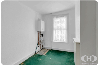
BOX ROOM / BOILER
