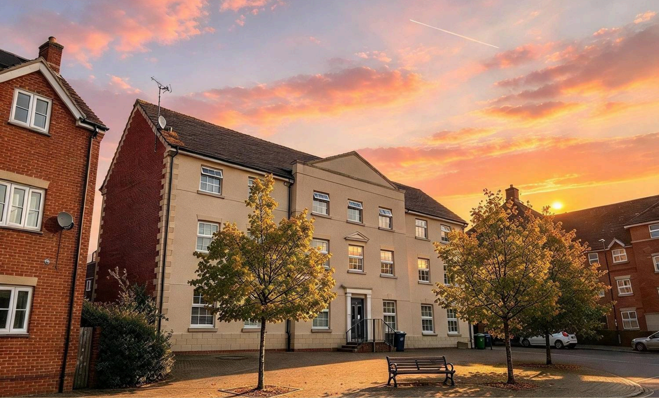
Bainton House, Millgrove Street, Bainton House Swindon
