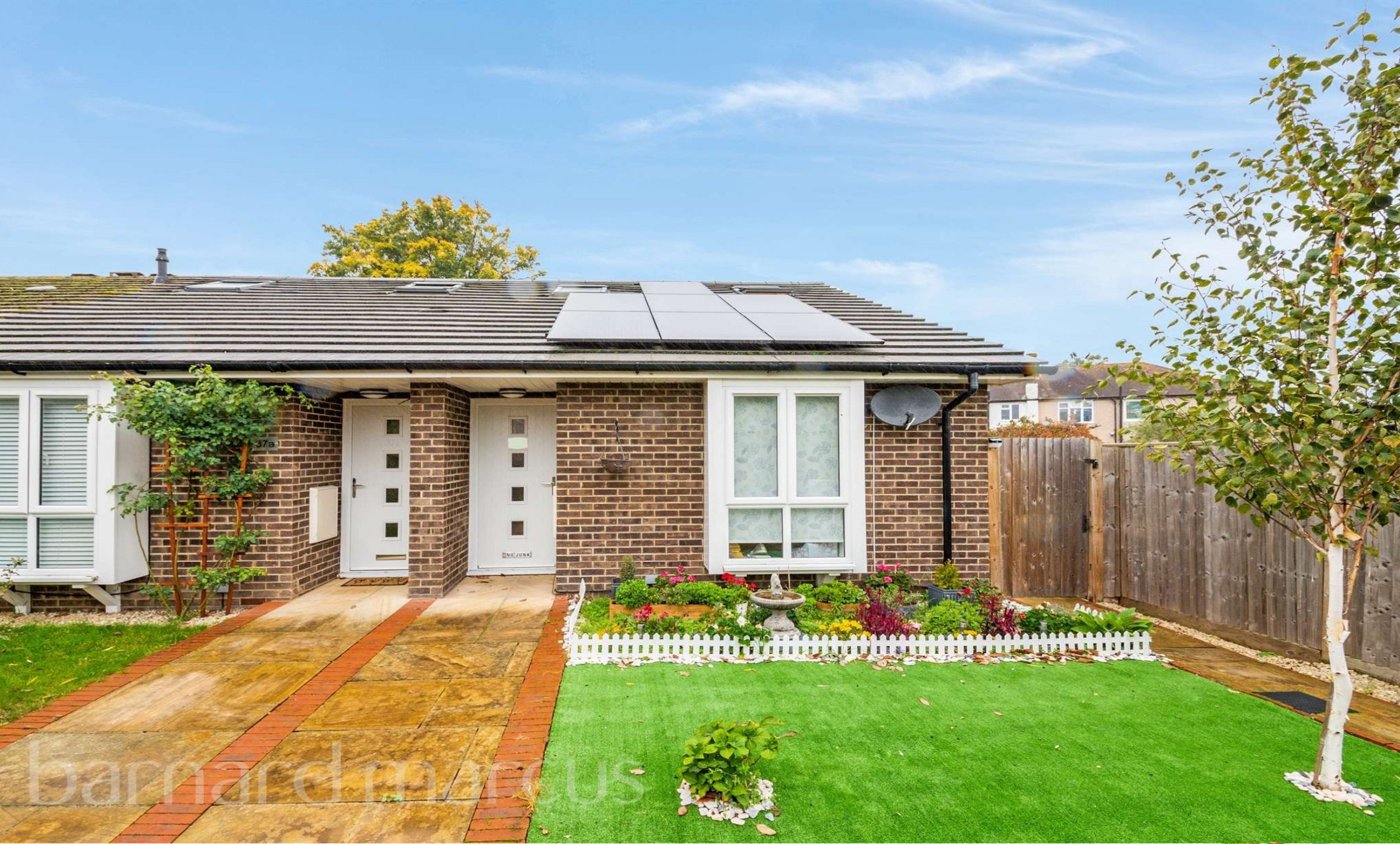
Southwood Close, Worcester Park, KT4 8QH
