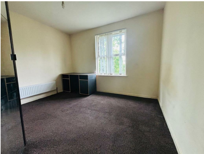
Double glazed window, central heating radiator
