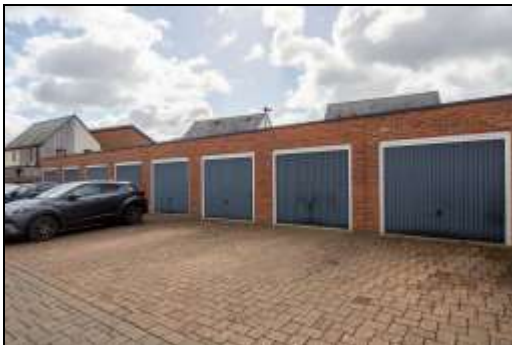
Garage in Block
