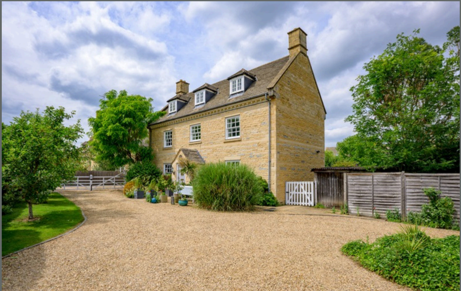
Orchard House Water Newton
