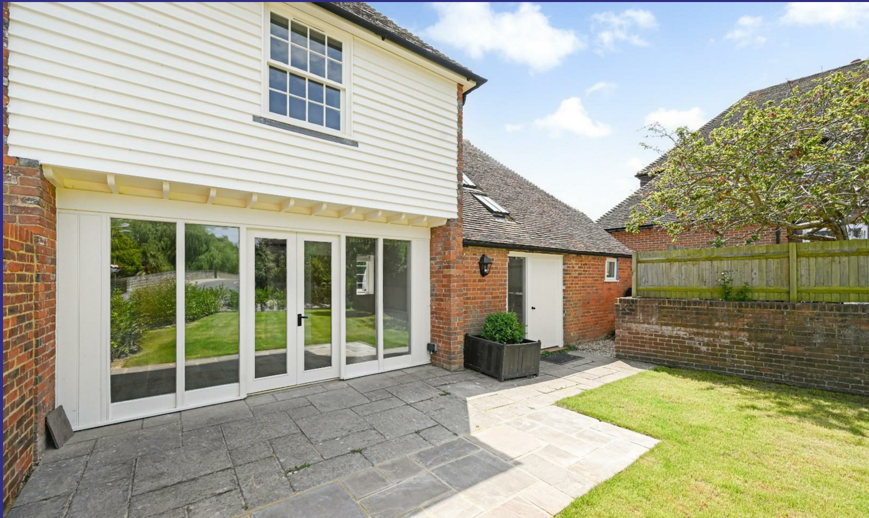
Bridge Street Wye
