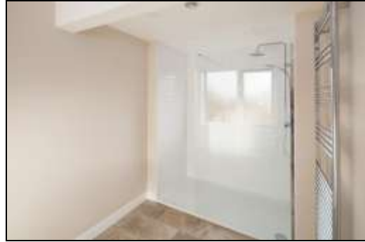
Re-Fitted En-Suite Shower Room
