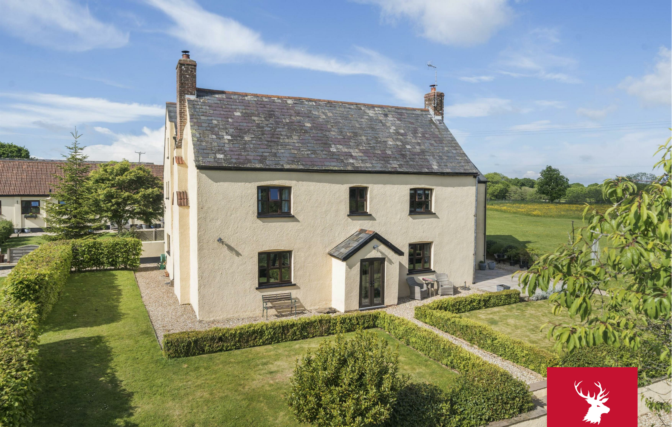
Lower Southbrook Farm, Southbrook Lane
