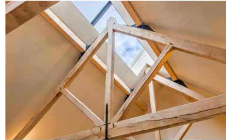
Ceiling of the Garden Room
