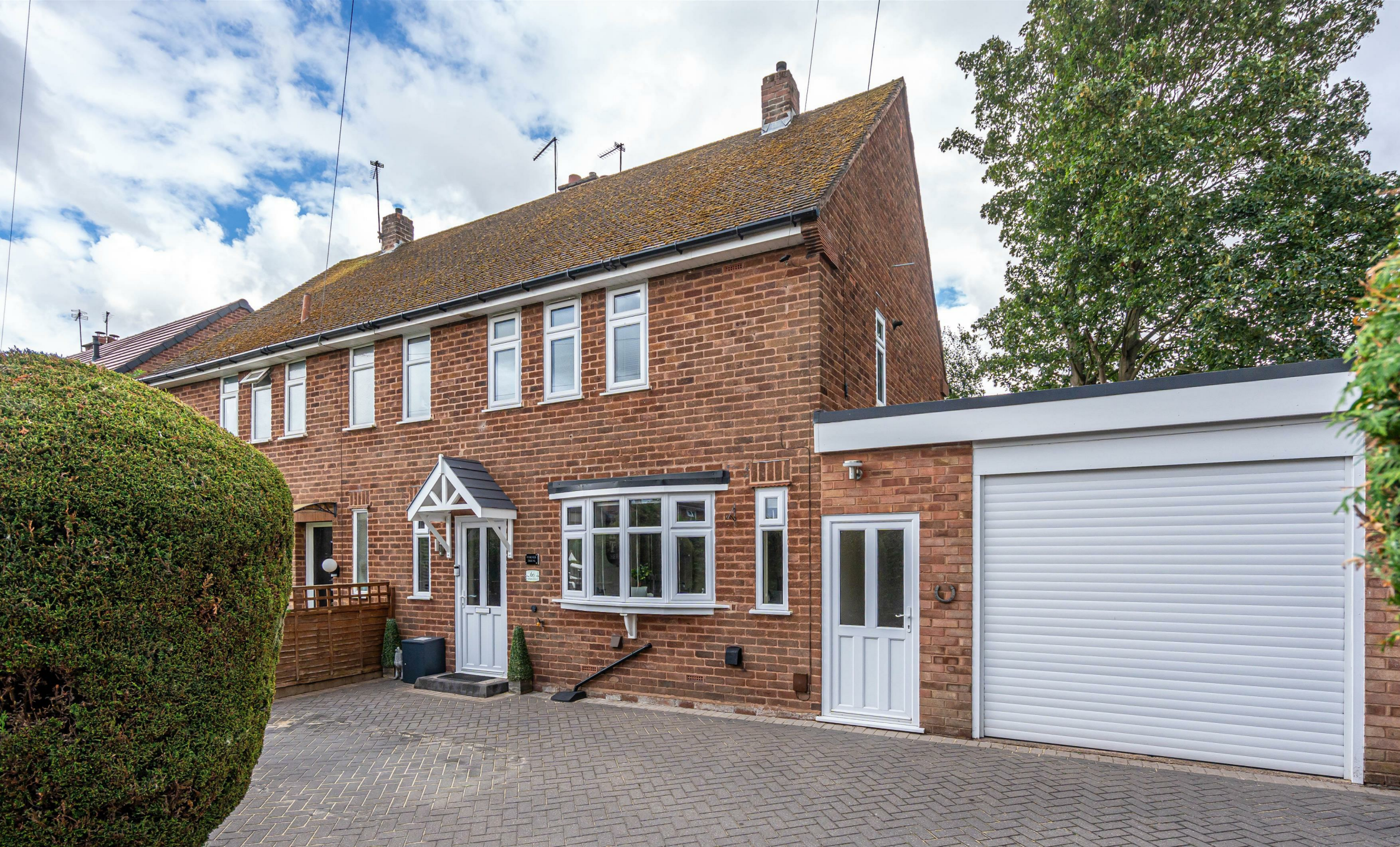
Corner House, 6 Palmers Way, Codsall, Wolverhampton, WV8 2JY
