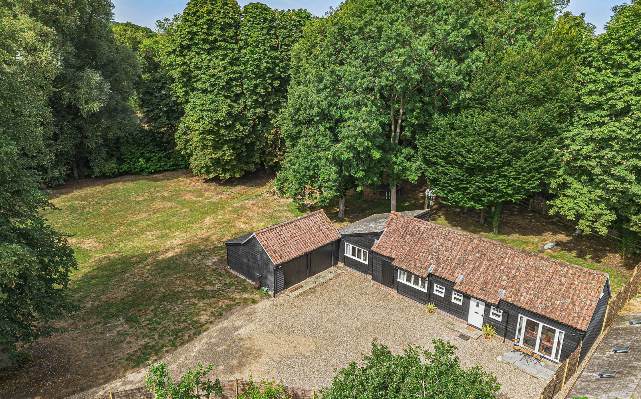
Three Hills Barn, Crossways House, Bartlow, CB21 4PW
