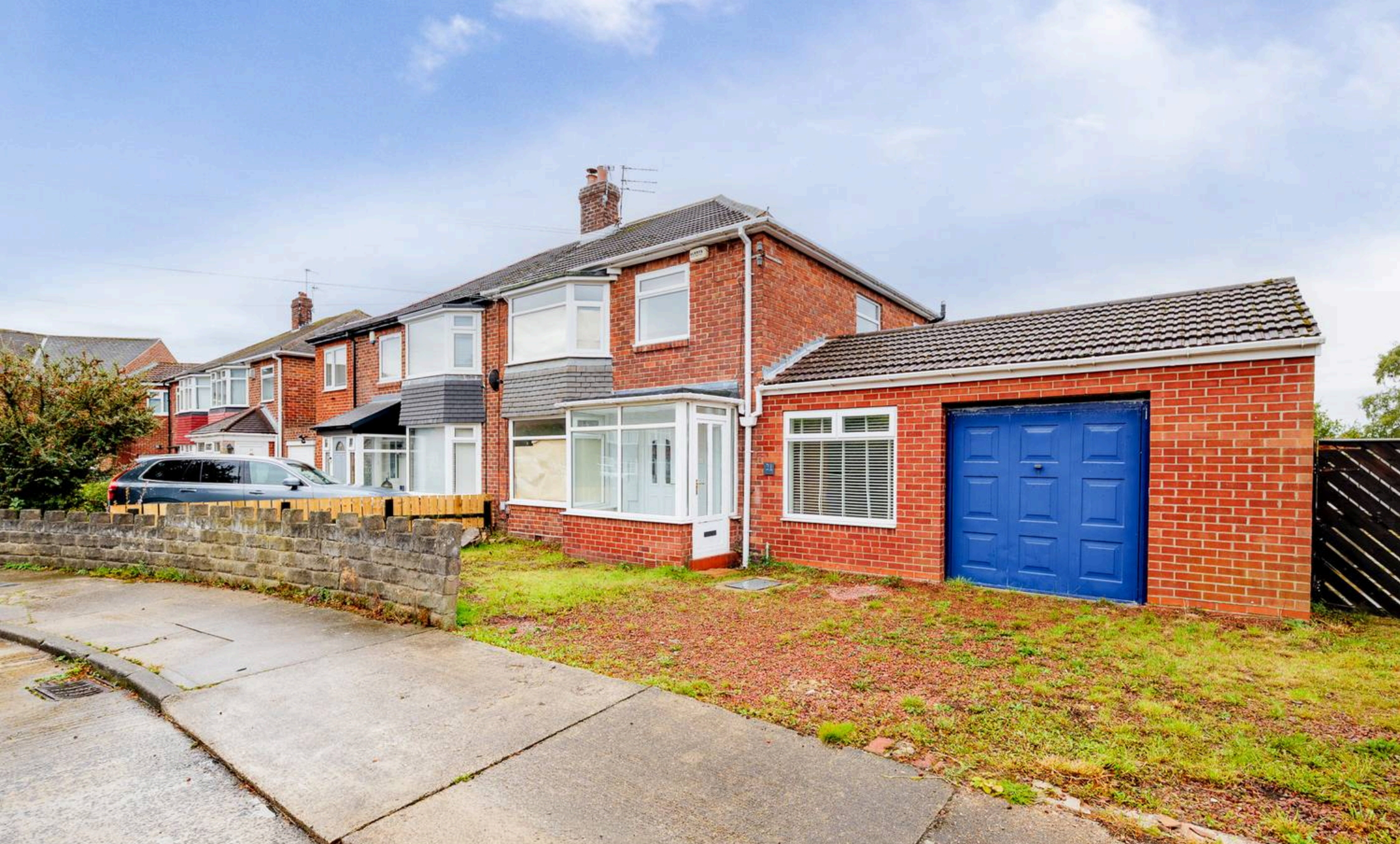
Dovecote Road, Forest Hall Newcastle Upon Tyne
