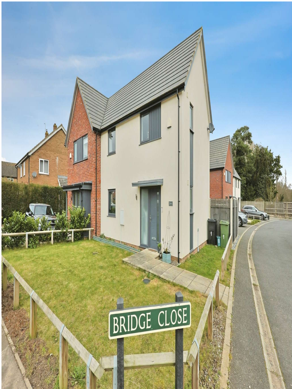
Bridge Close, Great Witchingham, NR9 5TE
