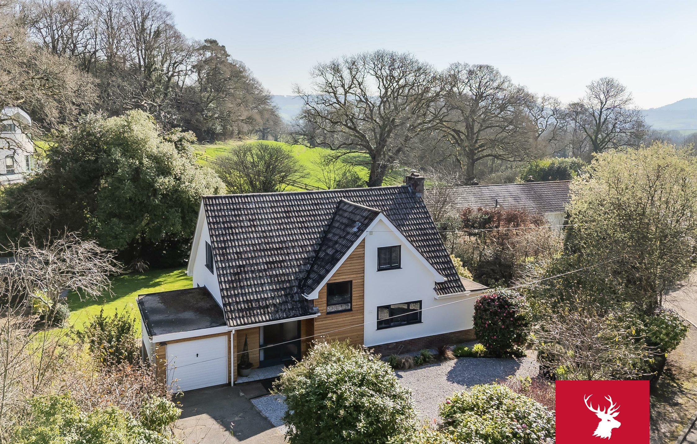
Timbers Lower Broad Oak Road
