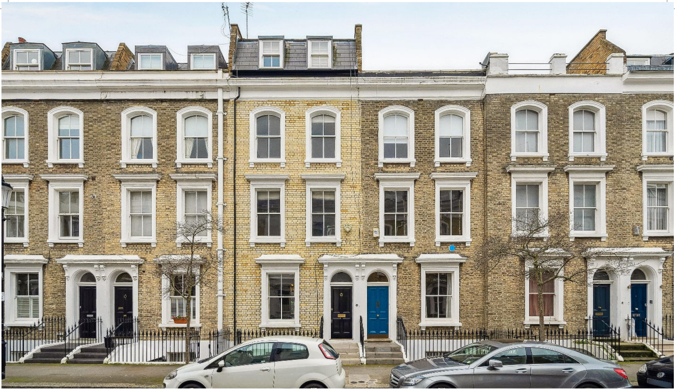
Ifield Road, London SW10
