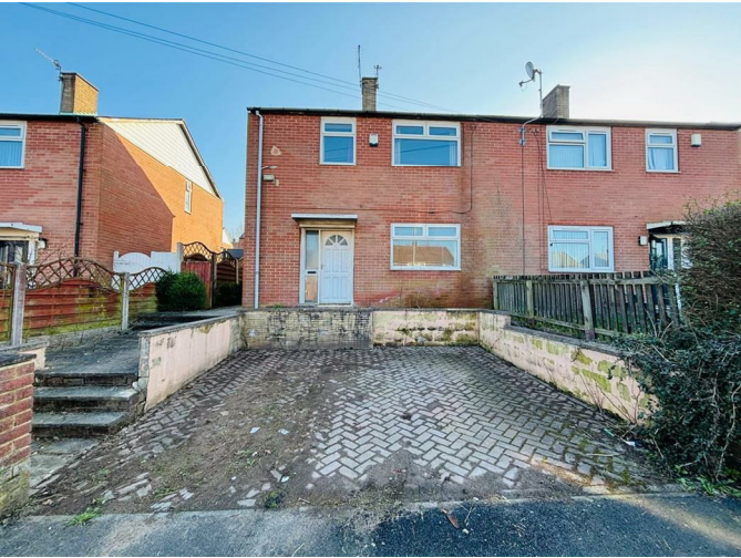
Off street parking to front
