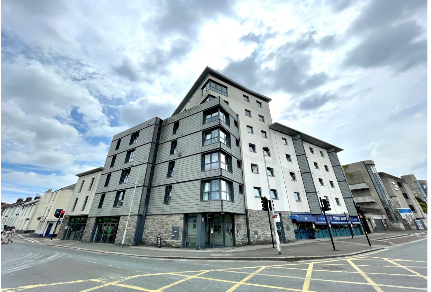
Penrose House, Lockyers Quay, East End Harbour, PL4 0DX
