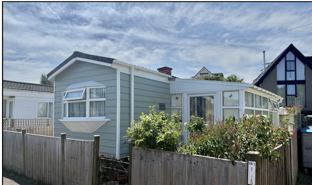
Single Unit Park Home close to Shops, Services & Transport Links
