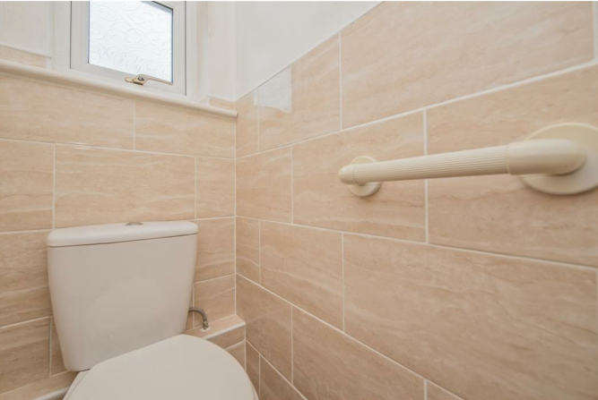
Double glazed window, low flush WC.
