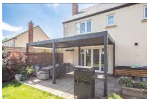
Pergola and Patio
