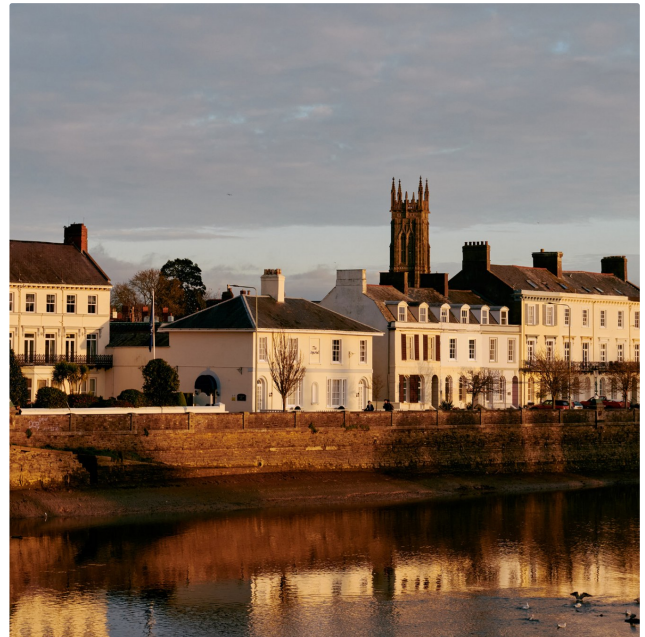
Taw Vale Parade at dusk. Nos. 7 and 8 sit within this terrace, directly above the river wall.
