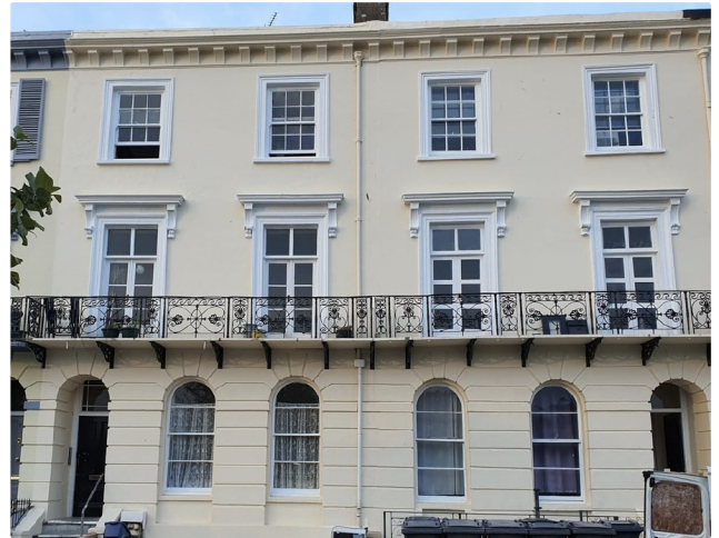
The front elevation, following external redecoration – original sash windows, arched ground-floor openings and the wrought-iron balcony that runs the length of the terrace.
