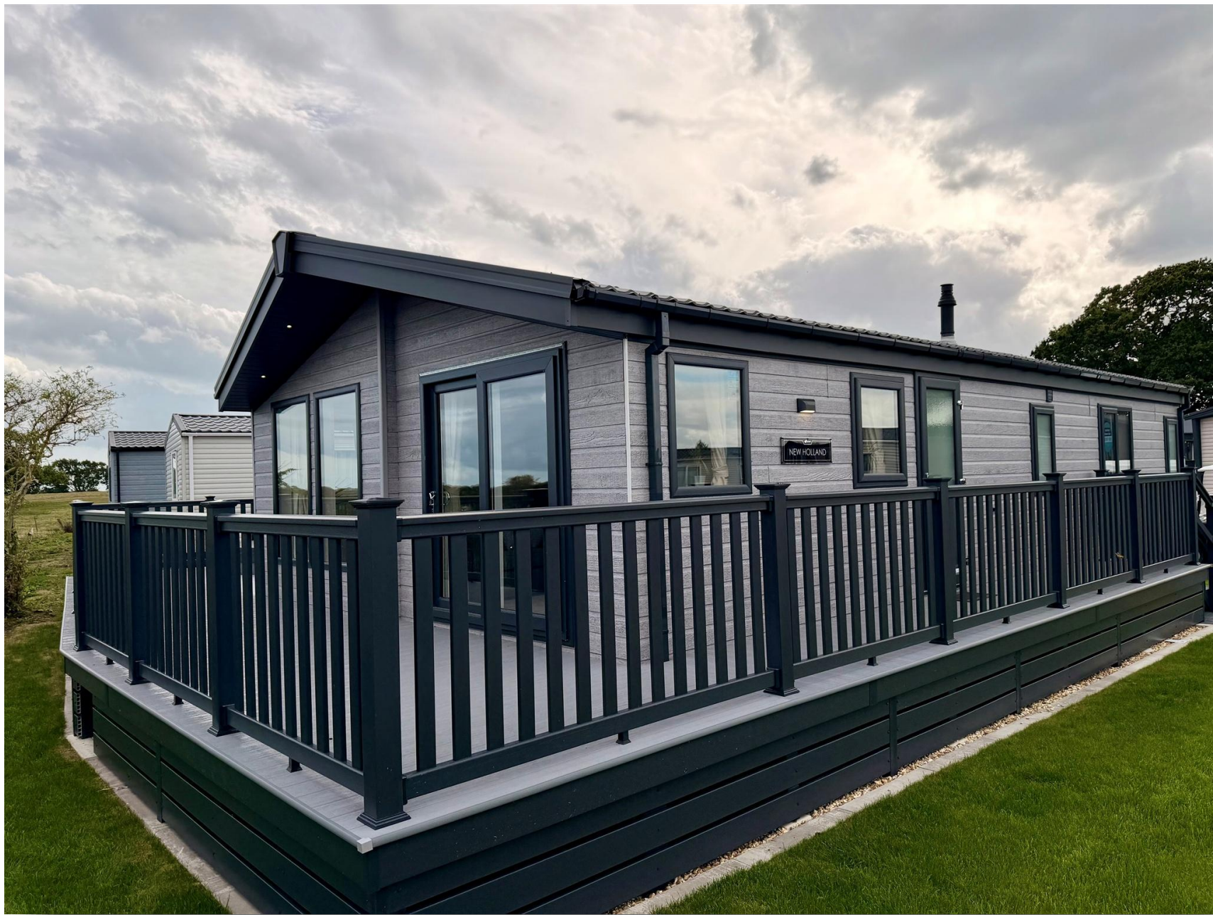
Holland Lodge, Mill Rythe Coastal Village, Havant Road PO11 0PB
