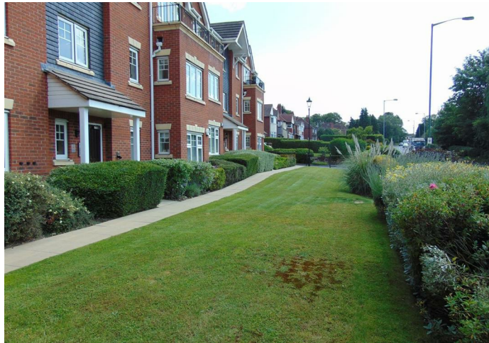
Well Kept Grounds
