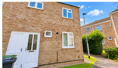
End terrace exterior
