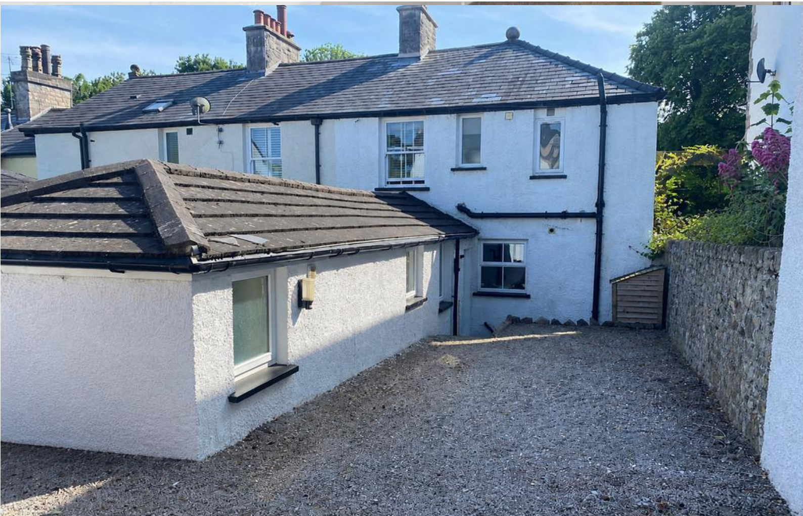
Rear Aspect and Courtyard
