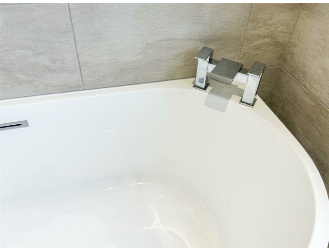
The Bathroom Finishes
