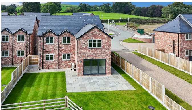
To the Rear of the Property
