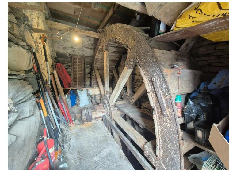
Located to the lower ground floor is the original water wheel, an impressive structure which interconnected with the mill pond still visible to the rear garden. Thereafter, the shaft leads through to the main mill where the original gearing is still in situ. It is an impressive sight with substantial supporting timbers, wrought iron ring gears and shafts which would have interconnected with the threshing room to the first floor. It has a stone floor in the main with high open
