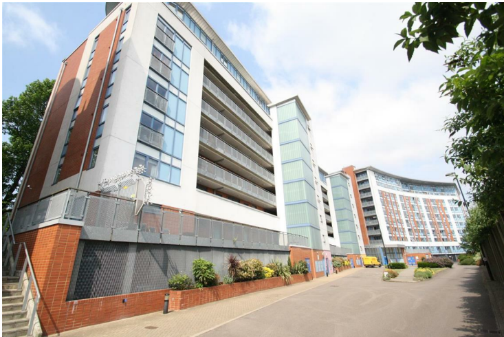
TAY COURT BUILDING VIEW
