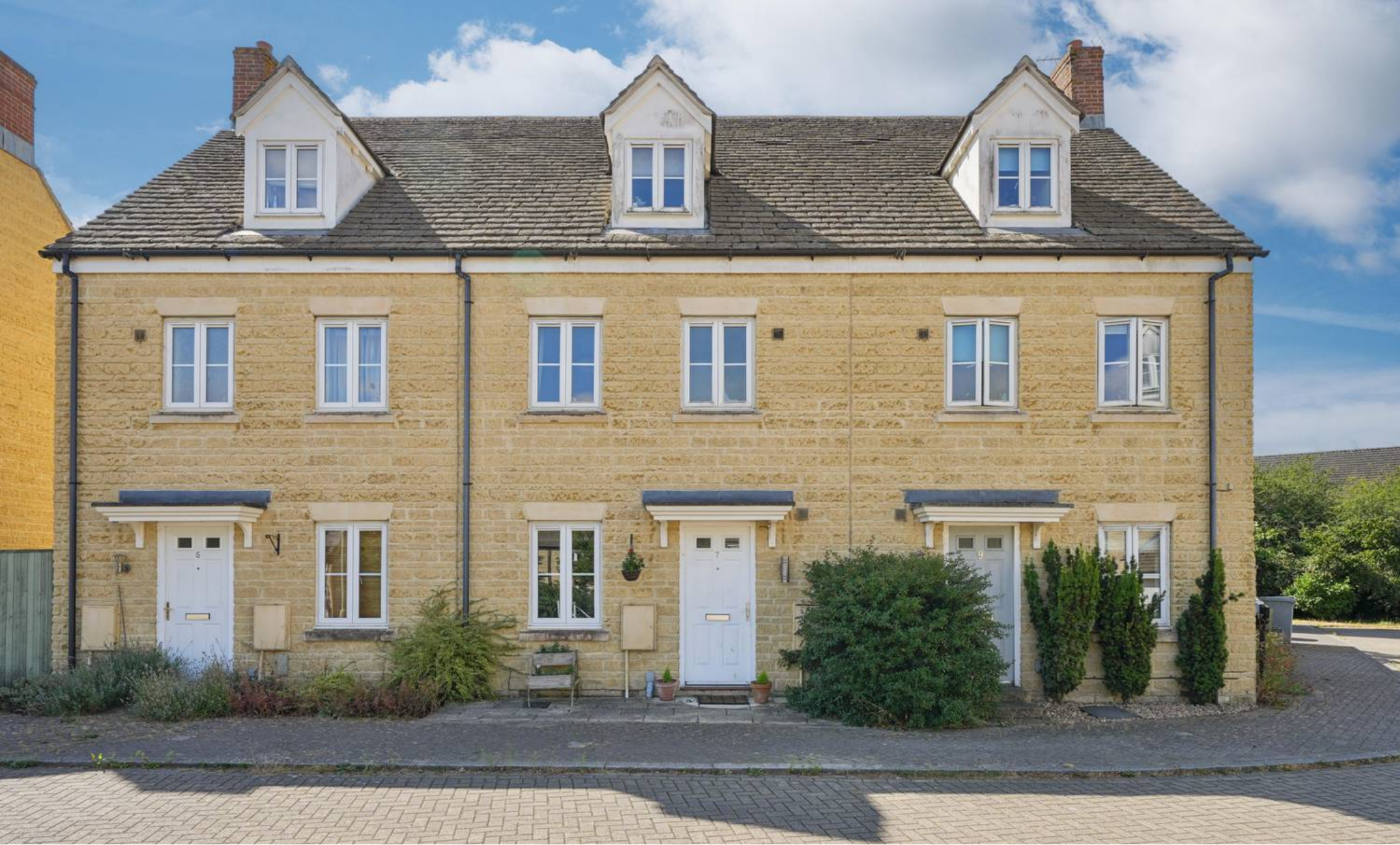
7 Northfield Road, Witney
