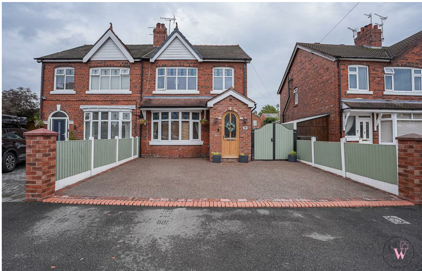
Tynedale Avenue, Crewe CW2 7NY
