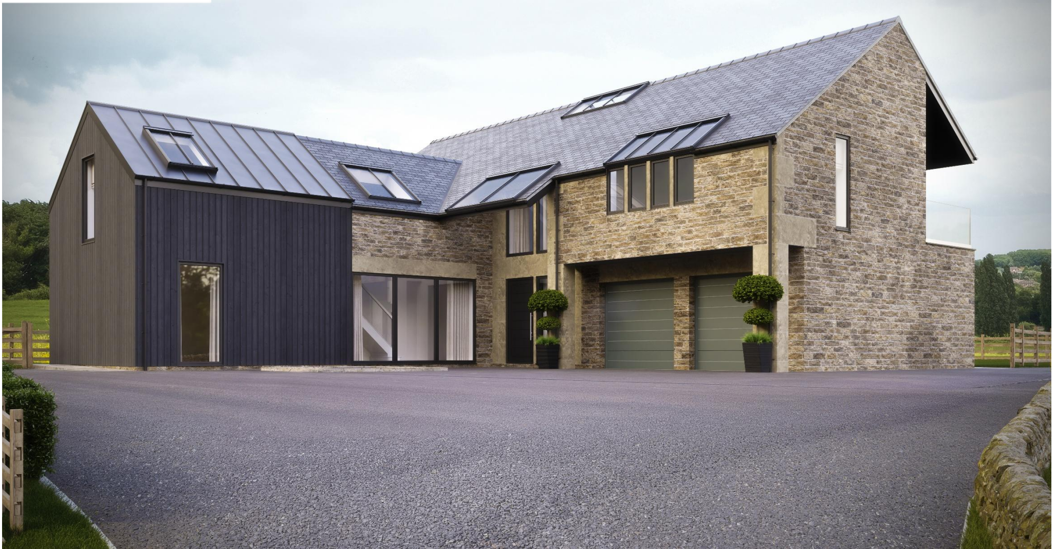
WEST VIEW HOUSE, BUILDING PLOT (4), HARDINGLEY FARM, SHELLEY, HUDDERSFIELD
