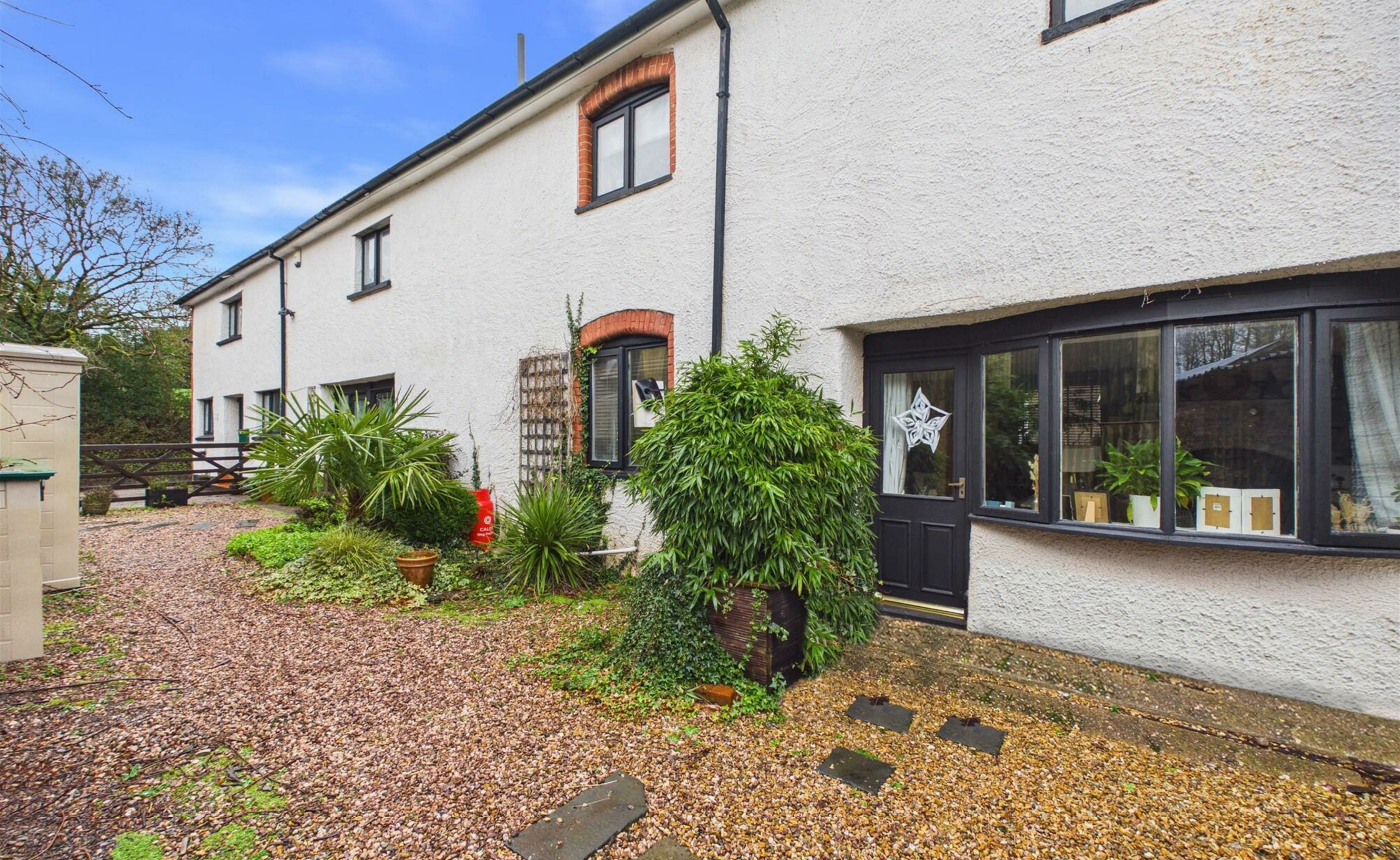
Burley House Silverton, Exeter, EX5 4HU £650,000
