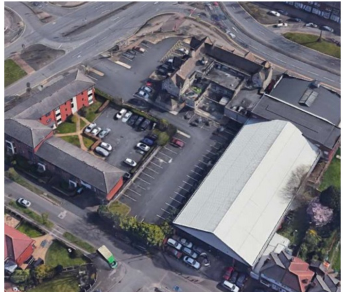
Aerial view of the site
