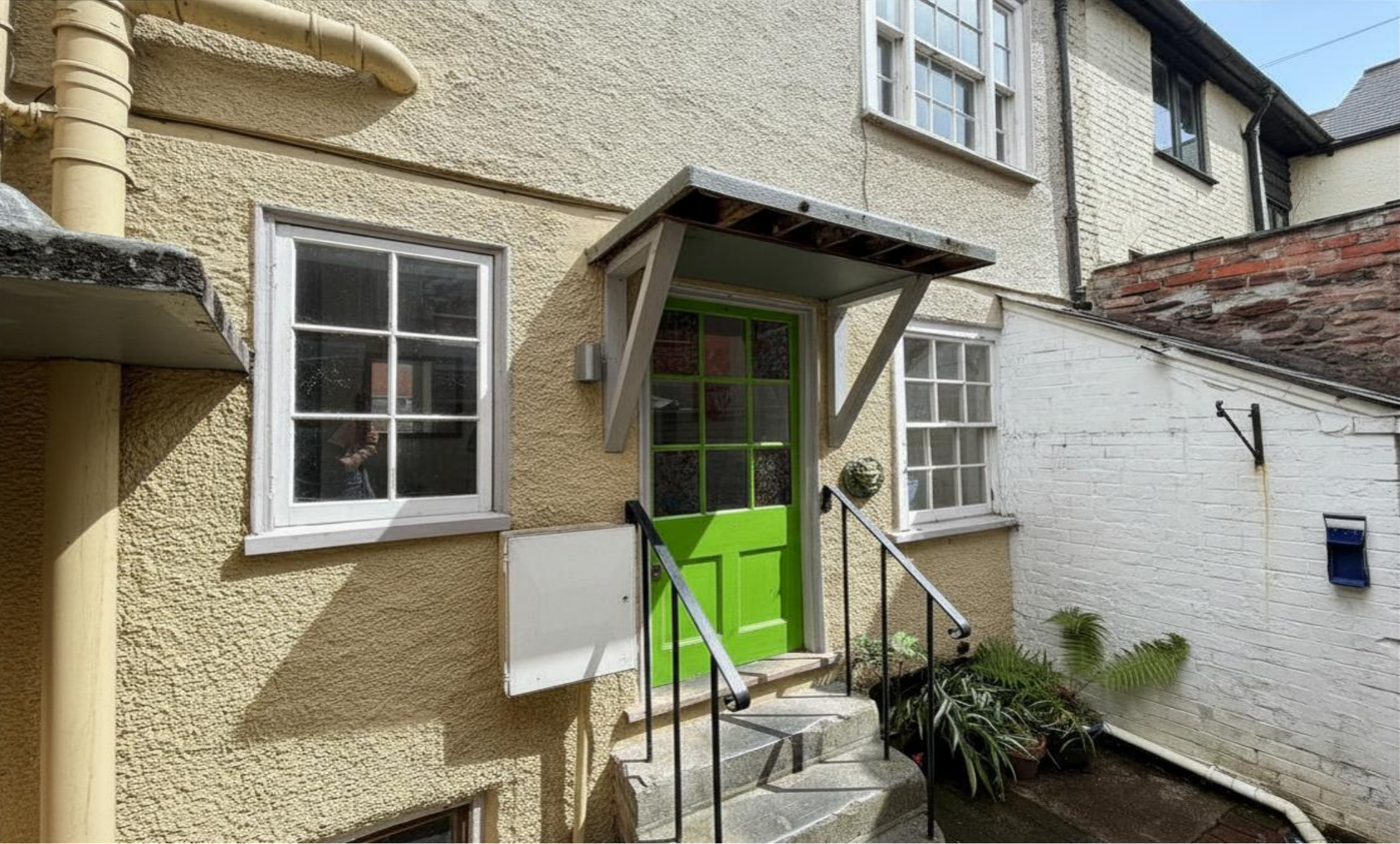
Radford Cottage, Barrington Street, Tiverton EX16 6PU
